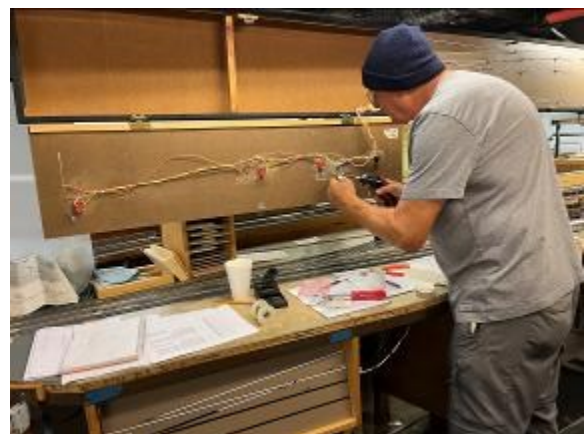
Bob Hanmer grabbed this photo of me putting on my Maintainer hat as I soldered the leads to the replacement toggle – and within half an hour the yard was back in business.
