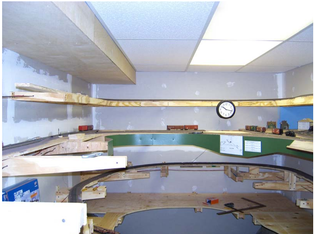
overview of the Tuolumne end of the room. The area to the left of the Tuolumne, in the foreground, will be the location of the Tuolumne WSLCo mill. In this view all four decks can be seen, from bottom to top - SP staging, Sierra mainline west of Chinese, Tuolumne and at the top the Pickering.
