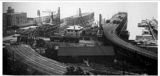
Fig. 8 – One of Erie’s covered piers under construction on the Weehawken riverfront – author’s collection
