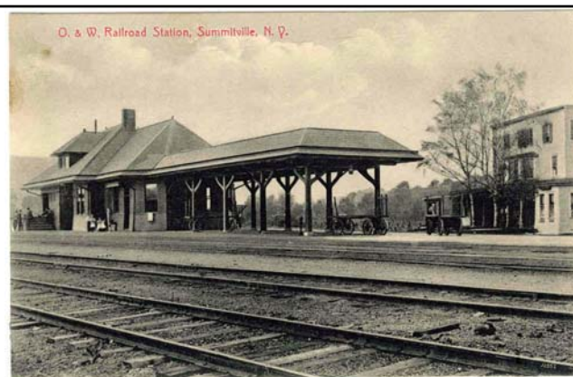
Fig 5: Summitville Station and Jones Hotel in 1913. The extended passenger canopy was added about a year earlier, providing shelter for the increasing number of passengers waiting to transfer between the Southern Division and Kingston branch trains. The Jones Hotel provided overnight accommodations, hearty meals and libations for weary passengers.– Author's collection
