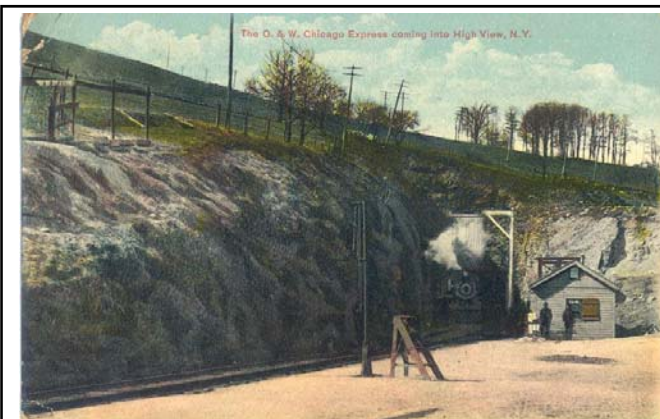
Fig. 11: A southbound train exiting Highview tunnel, soon to arrive at the station - Author's collection
