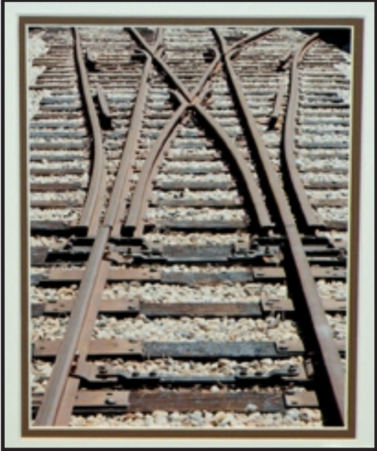
Bob Ziegler won First Place Photo "Track and Structures" category with his shot of a Stub Switch at the Nevada City Railroad Museum.
