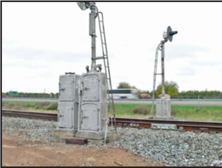
Searchlight Signals located at Fairmead are some of the last on the UP.
