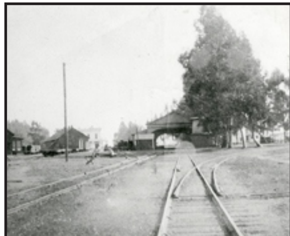
This view looks south from Thornton Avenue toward the SPCRR arcade-style station. The water tank is visible in the trees to the right/west of the station while the tracks on the right led to Dumbarton Point until 1880; after that year, the stopped at a wood yard near Ash Street for fuel for the locomotives. The Carter Brothers car shops are easily visible to the left of the station. - Collection Bruce MacGregor
