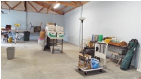
By 12-1-15 the interior had been insulated, walled, painted and lighted, and was ready for bench work.
