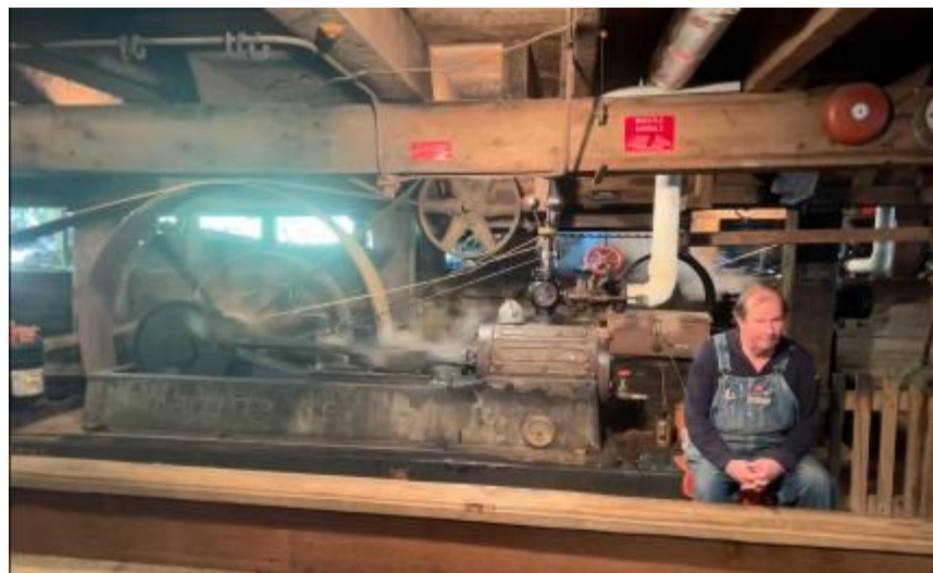
Under The Mill - The Main Sturgeon's Engine (and engineer)
