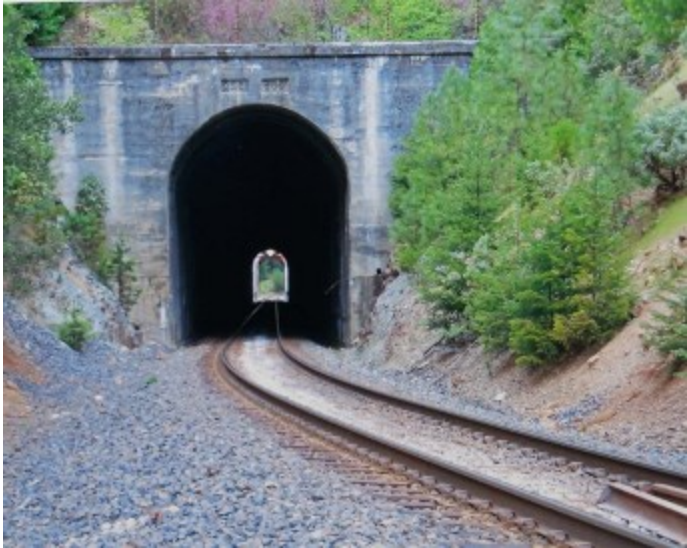
First Place, Photo, Track & Structures Walt Schedler SIMS Tunnel, Shasta Division
