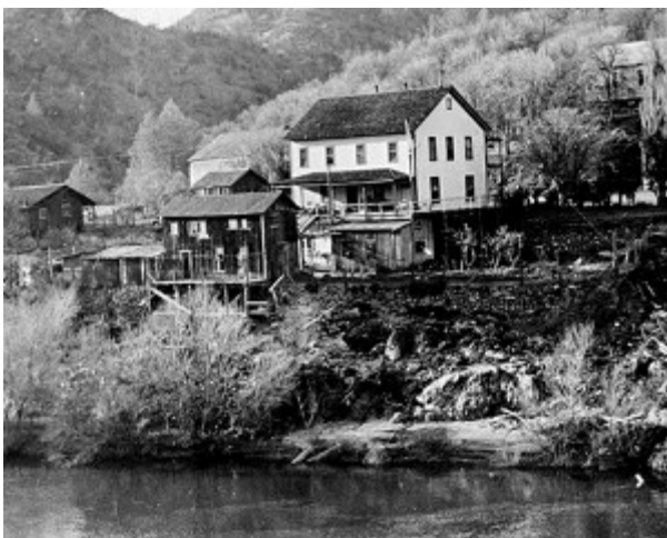
This is a very early photo of the Bagby Hotel with the Merced River on the foreground. The YVRR railroad tracks were on the other side of the hotel.
