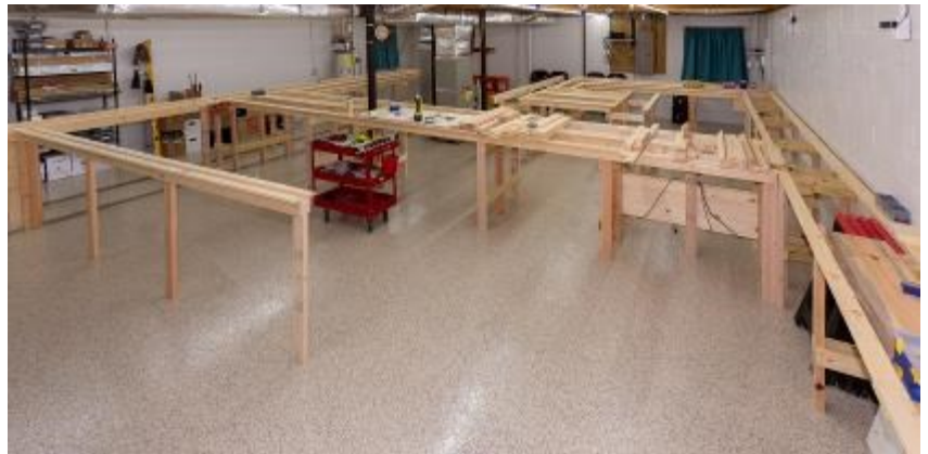
By the end of the first week of construction, 90% of the L-Girder benchwork was complete and installed.
