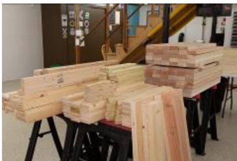
Legs, L-Girders, glue blocks, and cross members have been cut to size and are awaiting installation
