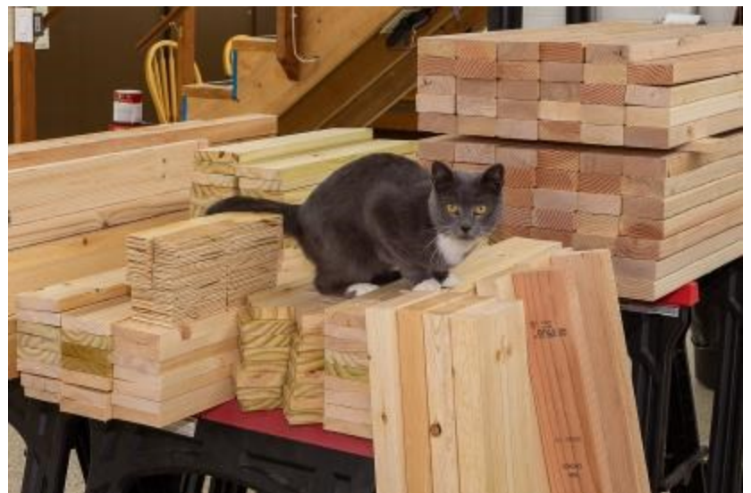
Meet Grigio, the newest member of the FMRR team. As Director of Quality Control, Grigio inspects the prefabricated assemblies
