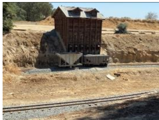
The Hillcrest and Wahtoke's ballast chute.
