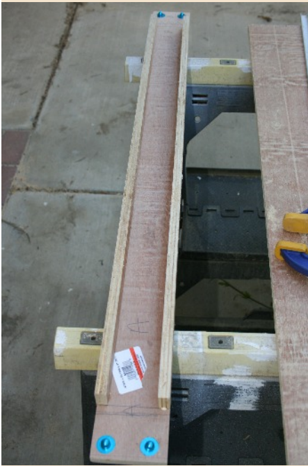
I added a flange to the underside of the lift-out gate for extra support
